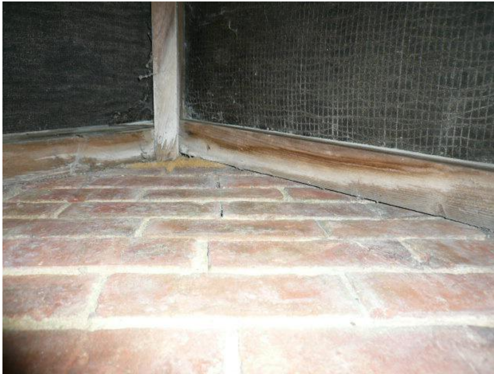
Photograph 6 The northern face of the central chimney
