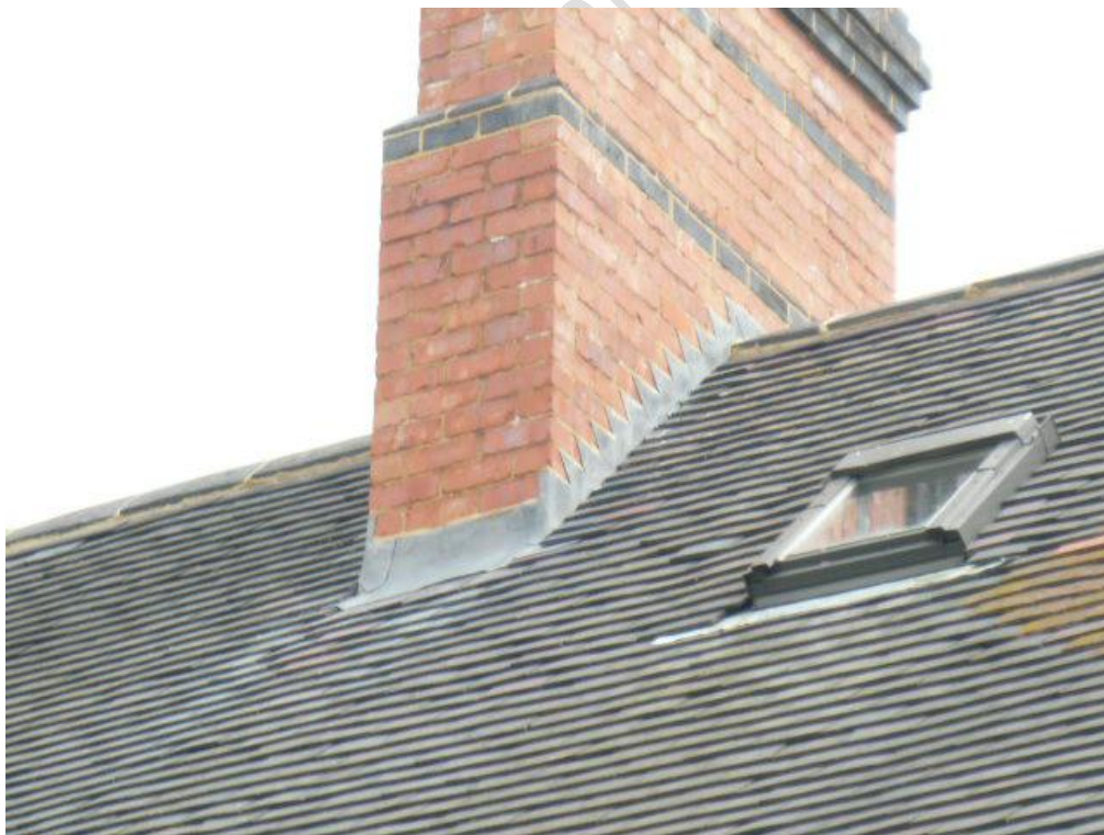
Photograph 3: The central chimney viewed from the South West
