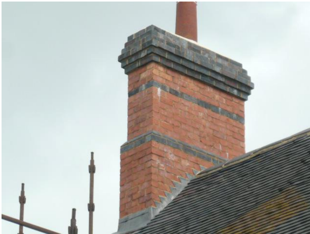
Photograph 2: The northern chimney viewed from the South West.
