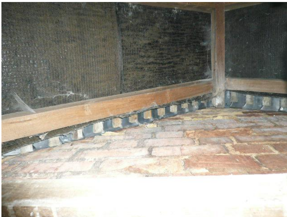
Photograph 7 The southern face of the central chimney
