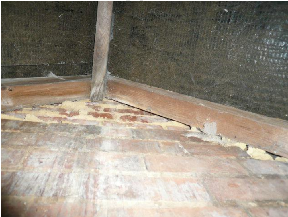
Photograph 5 The face of the North Chimney
